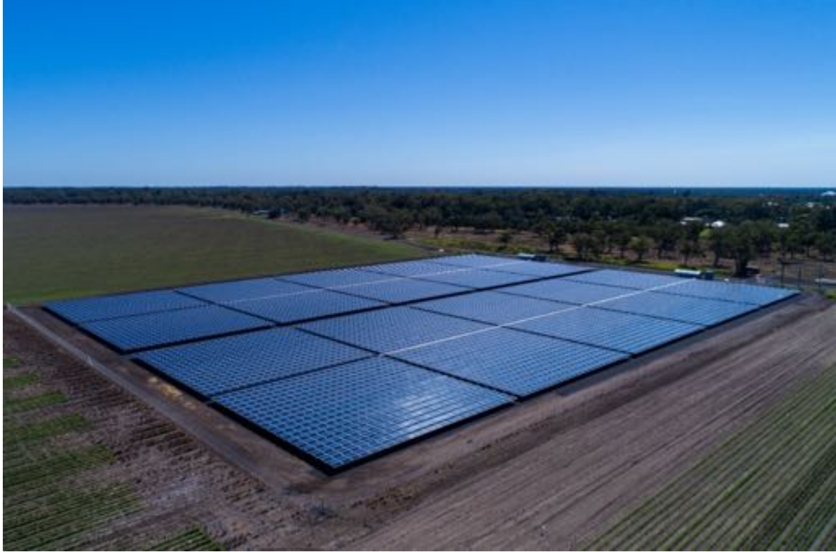
Chillamurra Solar Farm, Australia
