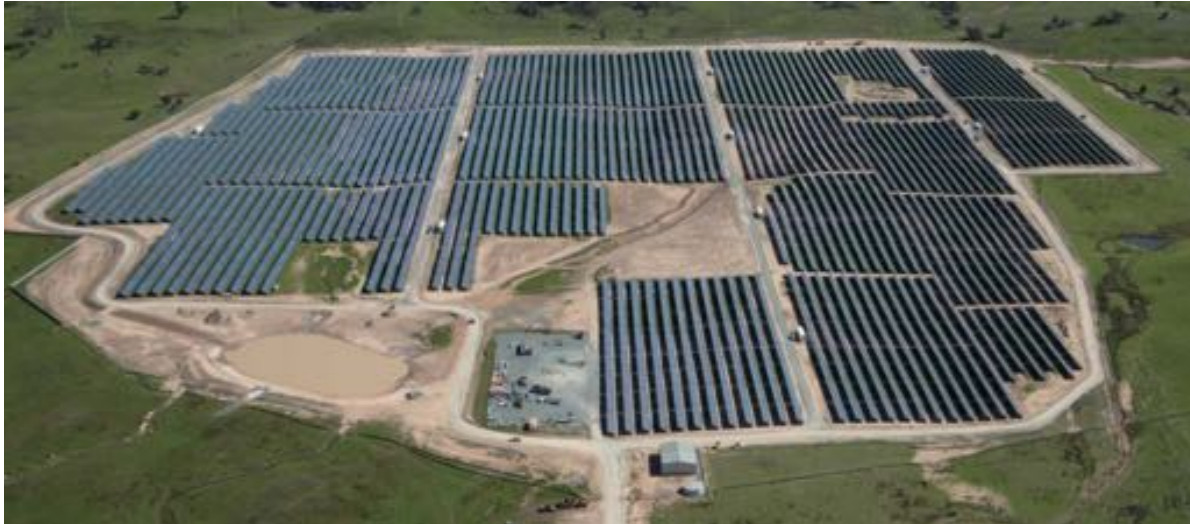
Royalla Solar Farm, ACT Australia
