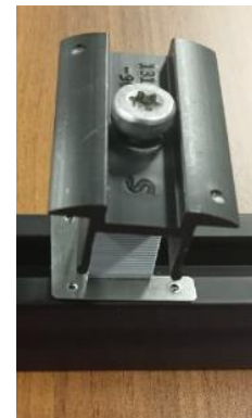
Fig 4.4.2A: Earthing Shim Alignment around mid-clamp
