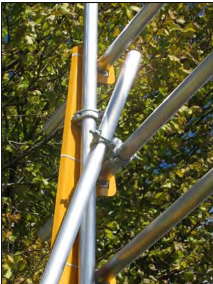
Raker/outrigger fixed to mid rail with swivel coupler.
