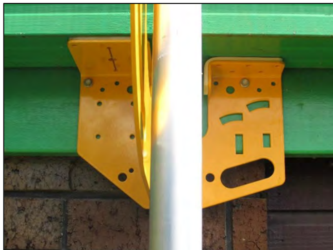
Multi bracket screwed in place correctly.
