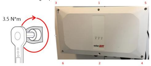
Figure 19: screw tightening sequence
